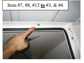
Continue around the entire kit bolting all **Ceiling** pieces to **Bulkheads** and **Doorframes** using ½ x ¾" carriage bolts, washers, and serrated nuts
